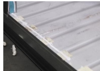
Figure 26: 1" Sika-Flex Bead on Floor
