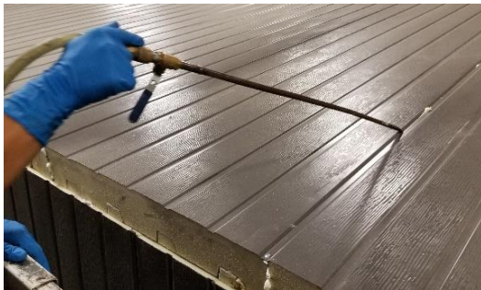
Figure 61: Removing debris from the roof panel joint
