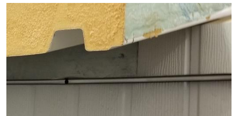
Figure 86: Installing Soffit J-Channel
