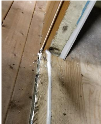
Figure 83: \frac{1}{2} " bead of Sikaflex 1A for sealing the threshold to the floor
