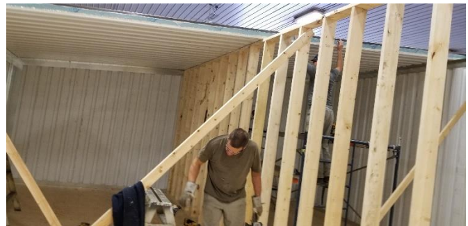
Figure 41: Temporary Support Wall with a mono pitch roof
