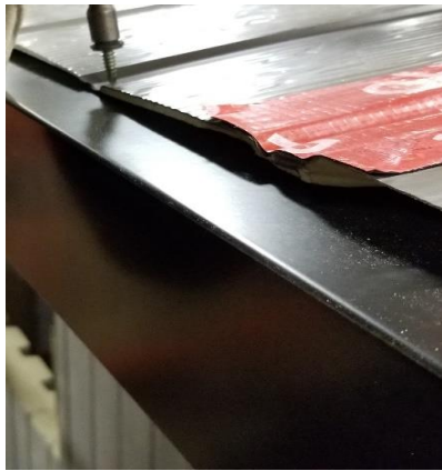
Figure 91: Drip edge fastened from the top in each panel recess
