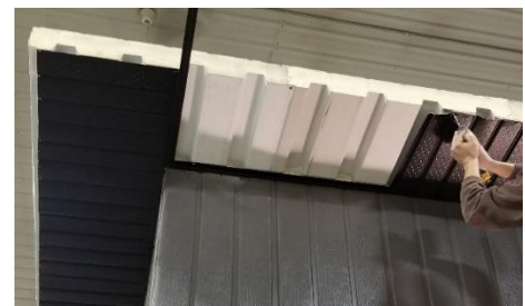
Figure 88: Installing soffit
