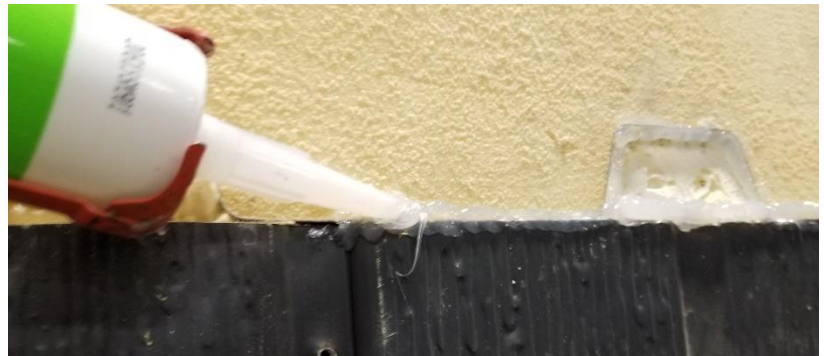
Figure 57: Sealing the roof panel to the wall and sealing the Foam Closures This must be done on roofs with or without eave overhang
