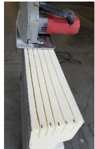
Figure 31: Narrow Panel Kerfs
