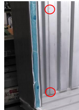
Figure 28: Screw Placement
