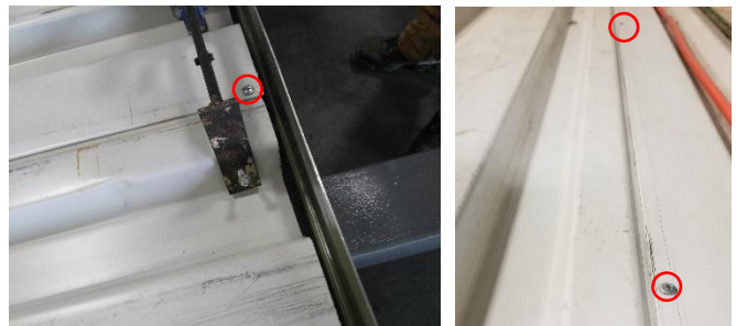
Figure 17: Pancake Head Screw Placement
