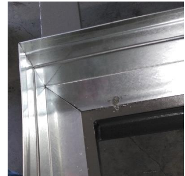
Figure 2: Mitered and Formed Corner
