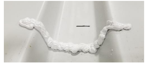
Figure 43: Foam Closures ½" Sikaflex 1A Bead
