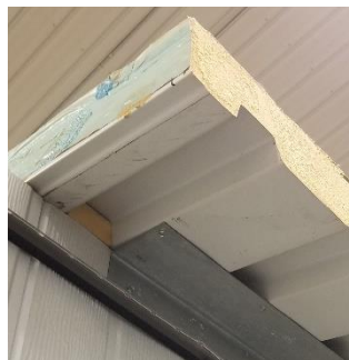
Figure 87: J-Channel with exterior angle installed
