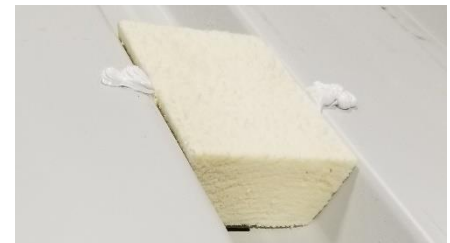
Figure 44: Installed Foam Closures
