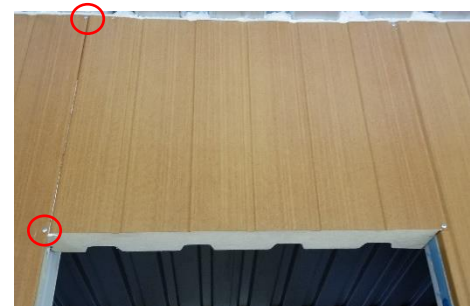
Figure 30: Screw Placement on Header Panel
