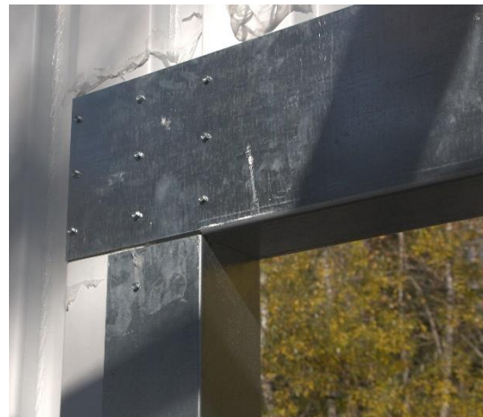
Figure 72: Header installed in garage door opening
