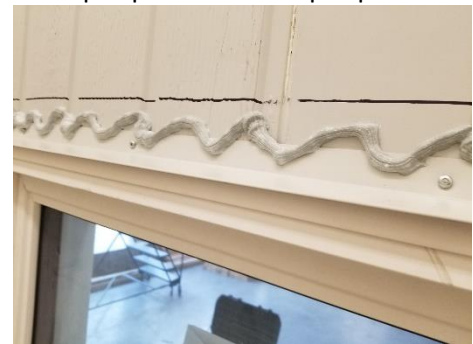
Figure 80: Serpentine bead of liquid flashing applied to drip cap
