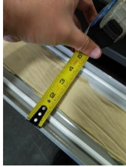
Figure 11: Sikaflex Bead Size ¼"
