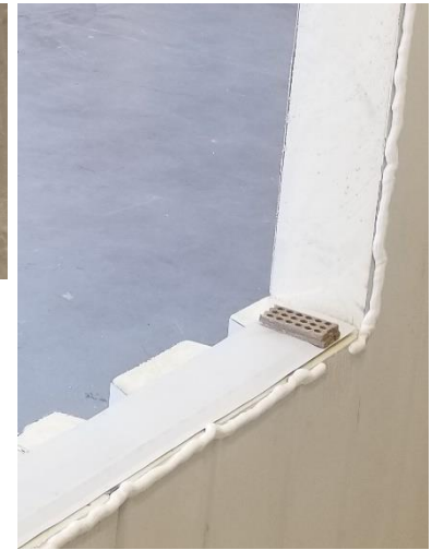
Figure 77: Sealant bead with drain gap
