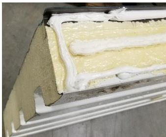
Figure 49A: Air barrier at the peak end, down the side and across the lower lip of the roof panel
