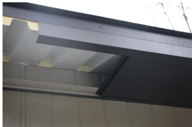
Figure 94: Fascia and Drip Edge installed prior to eavestrough installation
