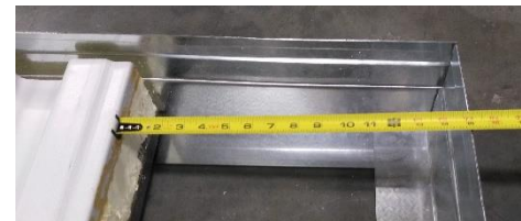
Figure 20: Last Floor Panel Measurement
