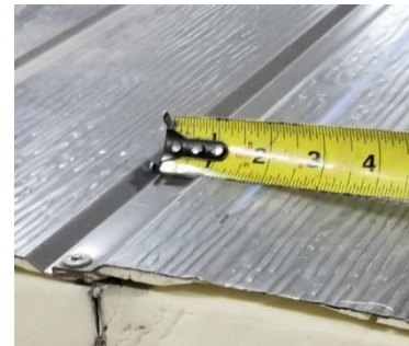
Figure 64: Snap a chalk line 2" from the seam.
