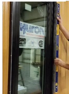
Figure 84: Ensuring the door is plumb and level before fastening
