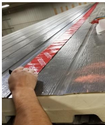
Figure 66: Aligning the barrier with the chalk line
