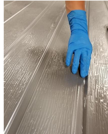
Figure 63: Working the silicone into the joint
