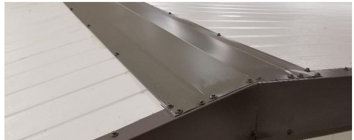
Figure 96: Colored stitch screws fastening the Ridge Cap
