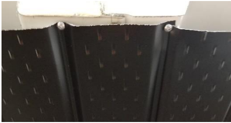
Figure 89: Fastening the Soffit
