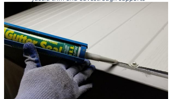
Figure 59: Sealing the roof eave kerf
