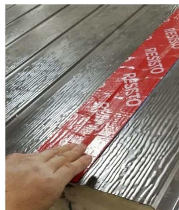
Figure 67: Applying the barrier
