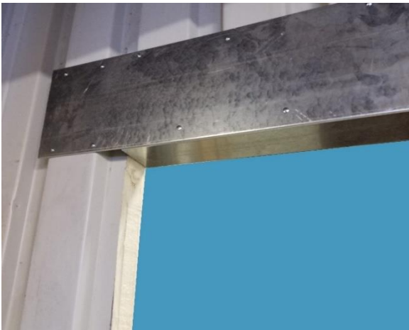
Figure 71: Header angle installed in window rough opening
