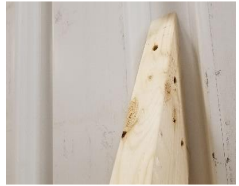
Figure 40: Top of Brace
