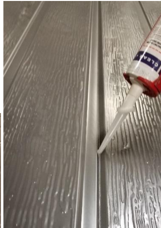
Figure 62: Applying silicone to the joint
