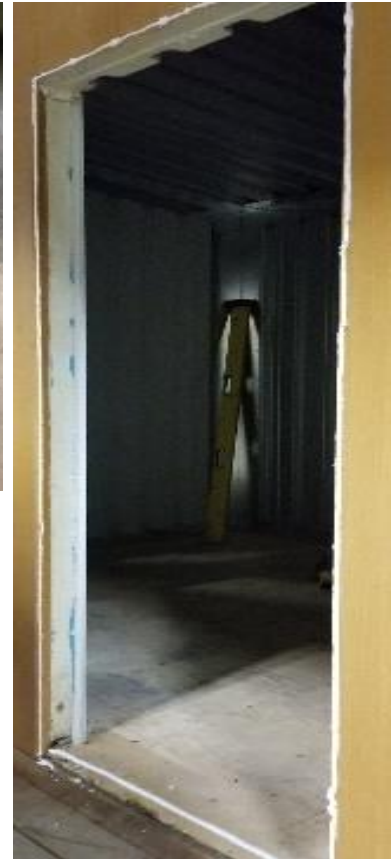
Figure 85: Sikaflex 1A bead around door opening
