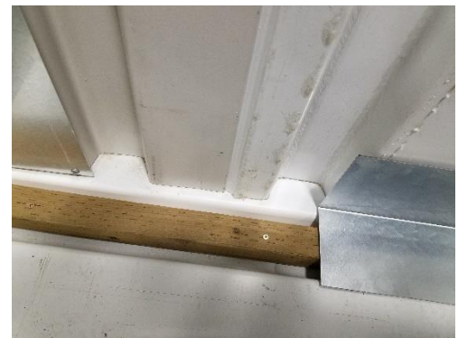
Figure 53: Structural lumber installed in flute above angle fastened with deck screws
