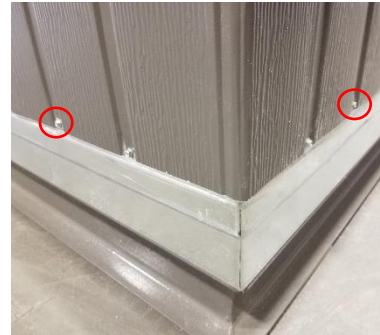
Figure 25: First Corner Installation
