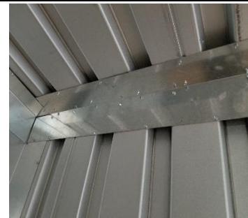
Figure 34: Floor to Wall Angle
